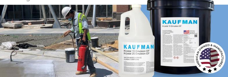
**Krystal 15 Emulsion EF** is a state of the art, water emulsion of 100% pure methyl methacrylate resin which produces a VOC compliant curing compound for curing, hardening, and dustproofing freshly placed concrete. Krystal 15 Emulsion EF provides total resistance to yellowing from ultraviolet exposure, is freeze-thaw stable, and due to the lack of any solvent odors, it is ideal for interior construction projects.
